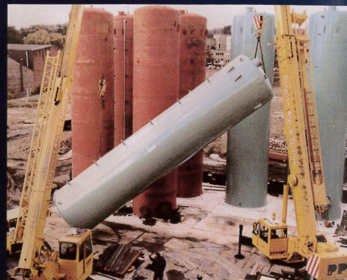
Offloading and positioning of 20 Wefco manufactured vertical 3m diameter storage tanks (photograph courtesy of Tetraosyl Limited).
